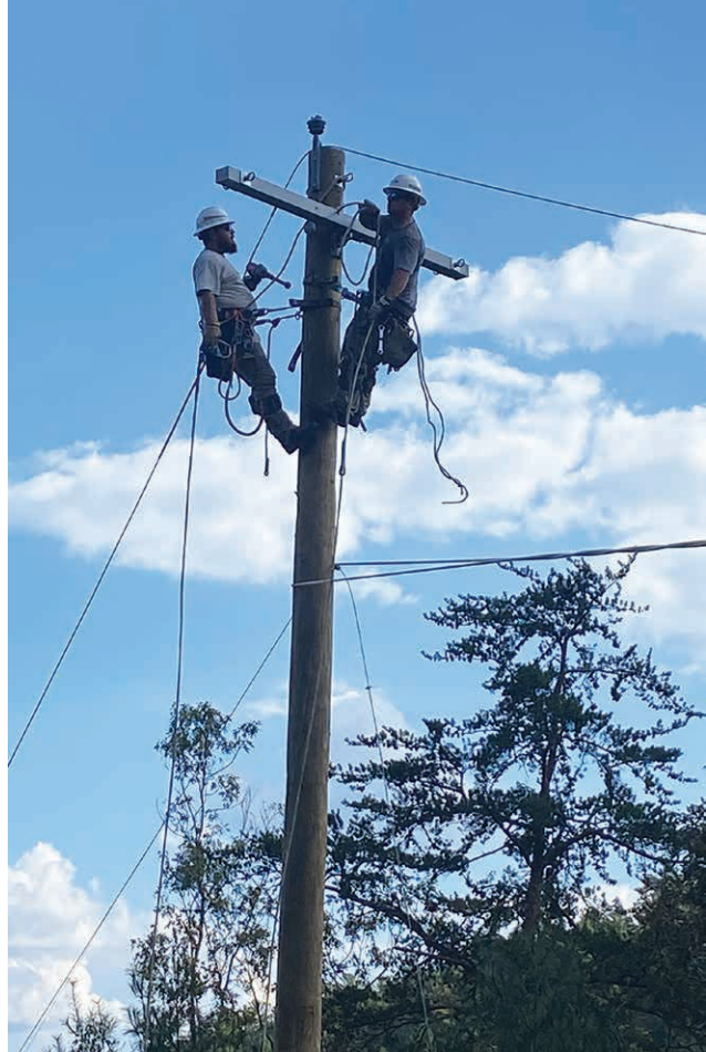
LEGWORK: Journeyman First Class Jake Strausbaugh, left, and Journeyman Second Class Ryan Gelnett re-string wire at the top of a pole.
