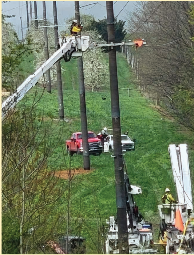
SYSTEM IMPROVEMENT: Adams Electric Cooperative has contracted AUI Power to set 15 ductile iron poles along the transmission circuit between the co-op's Orrtanna breaker station and its Fairfield substation. Above, AUI lineworkers make the final attachments to the transmission circuit while the lines are de-energized. The poles replace the original wooden poles set by the co-op in the early 1970s, which are starting to show animal, insect and weather damage. This section is the third of several sections that will be upgraded. To date, 47 of 97 poles have been replaced with the rest scheduled over the next three to four years.
