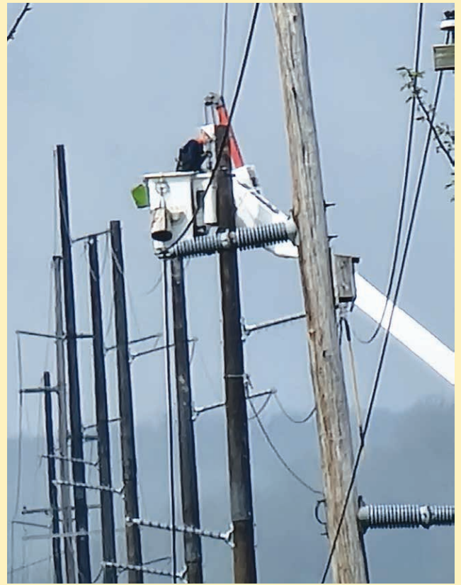
SYSTEM IMPROVEMENT: Adams Electric Cooperative has contracted AUI Power to set 15 ductile iron poles along the transmission circuit between the co-op's Orrtanna breaker station and its Fairfield substation. Above, AUI lineworkers make the final attachments to the transmission circuit while the lines are de-energized. The poles replace the original wooden poles set by the co-op in the early 1970s, which are starting to show animal, insect and weather damage. This section is the third of several sections that will be upgraded. To date, 47 of 97 poles have been replaced with the rest scheduled over the next three to four years.
