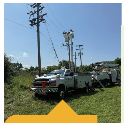
A Gettysburg crew replaces primary metering in Adams County during routine maintenance.
