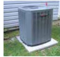
**Air-Source Heat Pumps:** During cold weather, an air-source heat pump absorbs heat from the air outside and transfers it indoors. During warm weather, the pump extracts heat from inside a building and pumps it outside. Heat pumps are especially efficient in spring and fall, when there may be a need for both heating and cooling comfort.
